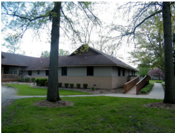
Rest-a-while "hotel" with handicapped entry
