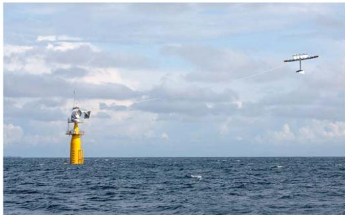
Floating wind turbines already exist, but they are unusable in many ocean areas because the water is too deep. The new technology, which uses a kite-like design tethered to a buoy, could dramatically expand the potential for offshore wind-power generation. Makani, the company behind the tests, says the deep-water turbines could eventually supply electricity to hundreds of millions of people.
