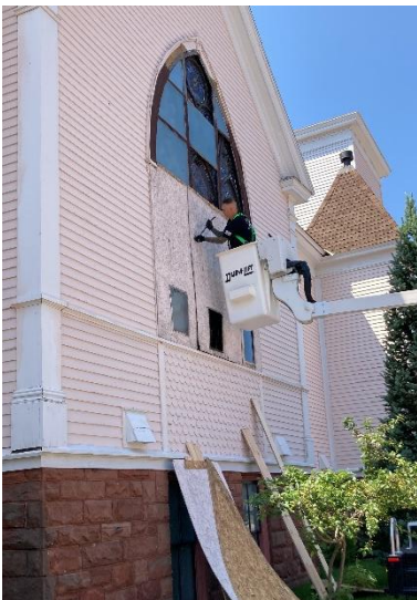
Protective particle board removed from one of the stained glass windows.
