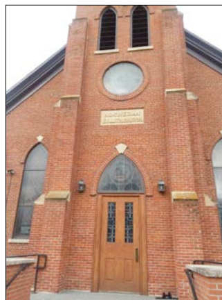
Norwegian Lutheran church originally built in 1876 in nearby Coon Valley
