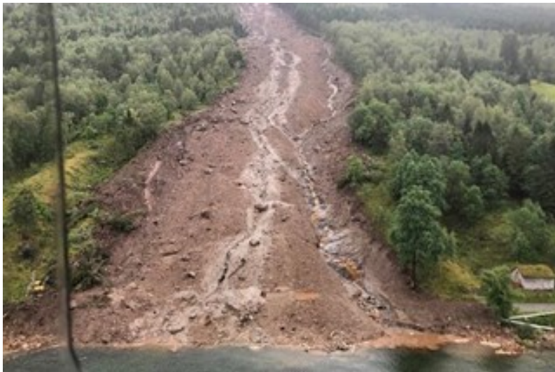
A landslide in July 2019 completely covered a rural road in Jølster, Norway. HRS SØR-NORGE
